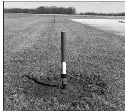
Blue reflectors like this will be replaced with new electric lights.
